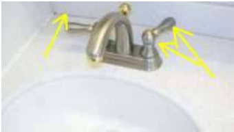
Photo 66-1 Disregard arrows showing damaged handle
