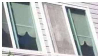
Photo 85-2 Damaged Window Screens
