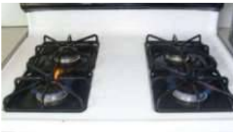
Photo 59-1 Two burners in front were only working
