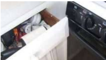
Photo 63-1 Cabinet door hitting stove
